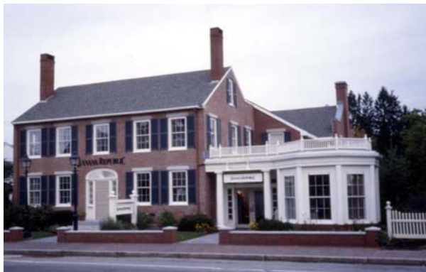
This Banana Republic clothing store in Freeport is designed to look like a house. A building like this in the Gateway district would be compatible with Pottstown's traditional neighborhoods.
