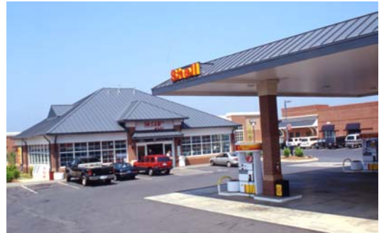
This convenience store, with an island for dispensing gasoline, is built of brick, with a standing seam hip roof, making it compatible with traditional neighborhoods.
